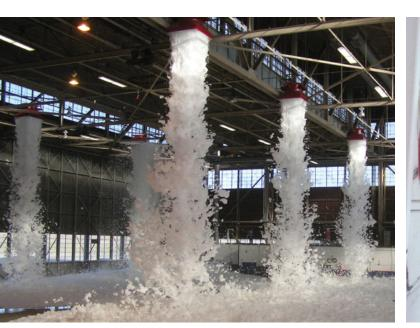
JET-X foam systems provide fire suppression solutions for a multitude of special hazards. The portfoilio offers UL Listed, FM Approved configurations, design flexiblity for utilization of inside or outside air supply, and specific generator models for LNG hazards. All JET-X generators are CE Marked in conformance with the Machinery Directive 2006/42/EC.
